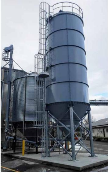
The end-user required additional storage capacity of wood pellet fuel used to fire a community boiler. The new system provided an extra storage buffer of the product when the supply of fuel to the site over the cold months became unreliable. The project scope was turnkey and included design, construction, and site installation of the silo and screw conveying system. Also included was the foundation design and build, electrical, and automation.
